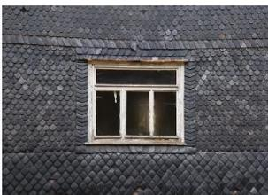
Figure 19 Slate shingles as wall finishing in historic buildings
